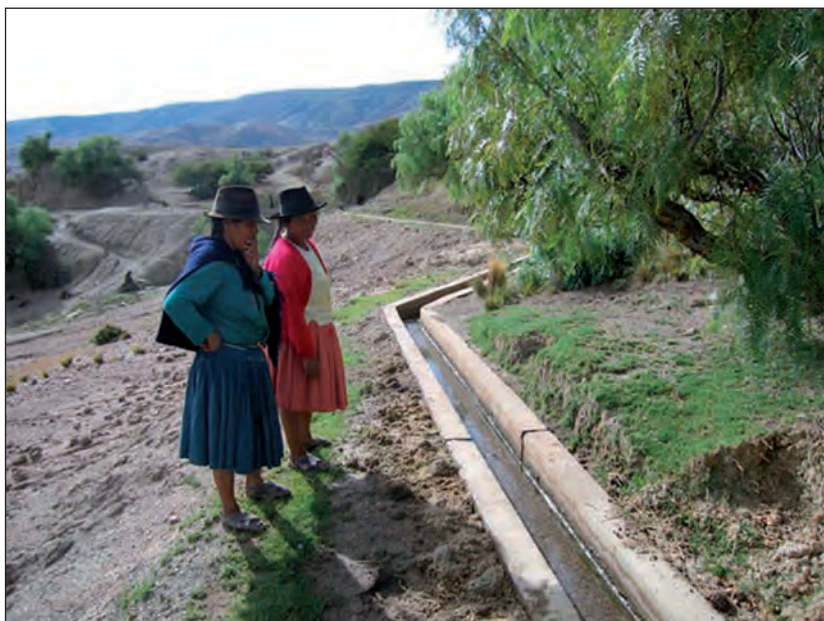
Figure 19 An irrigation channel in Bolivia
