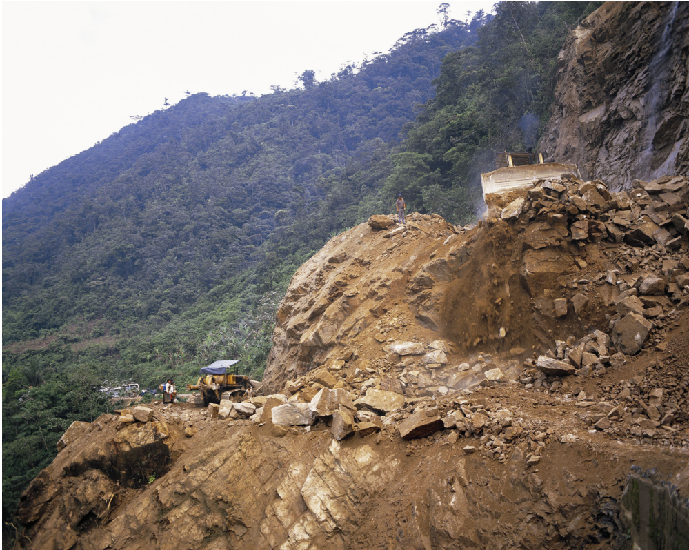
Landslide damage to a highway in the Andes
