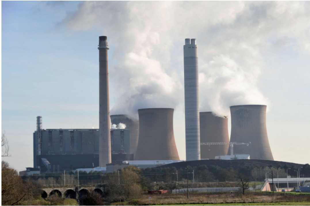
A coal-fired power station, Rugeley, Staffordshire
