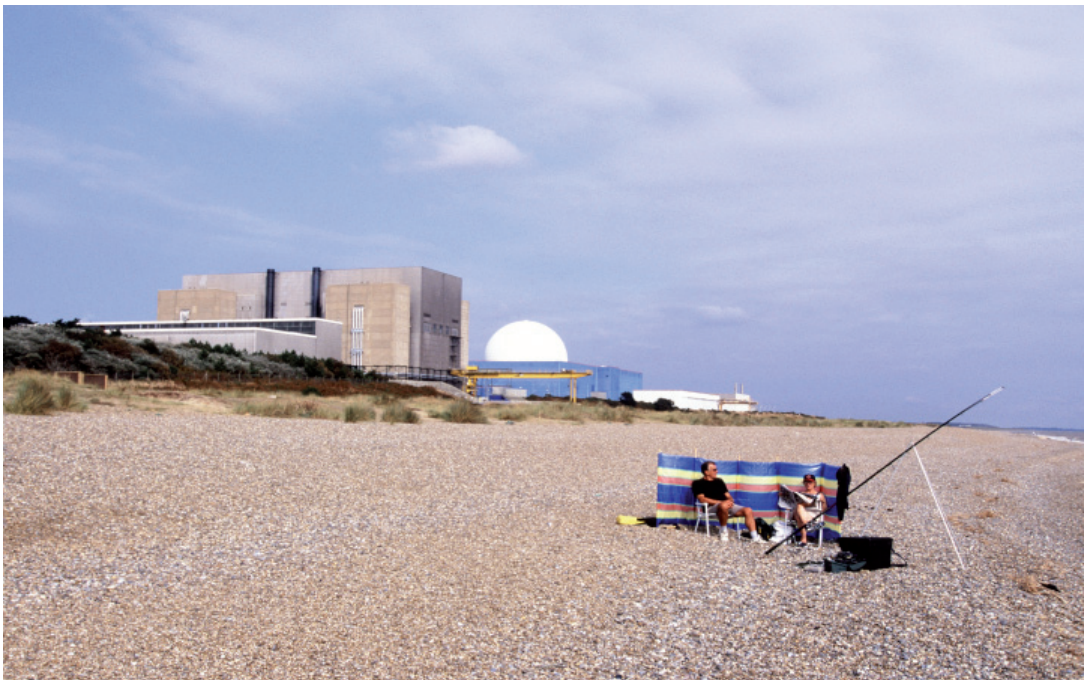
A nuclear power station, Sizewell, Suffolk
