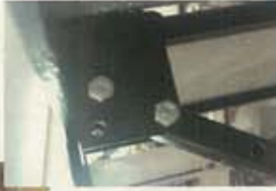
Top bracket with the back leg secured with M6 bolts and nuts.
