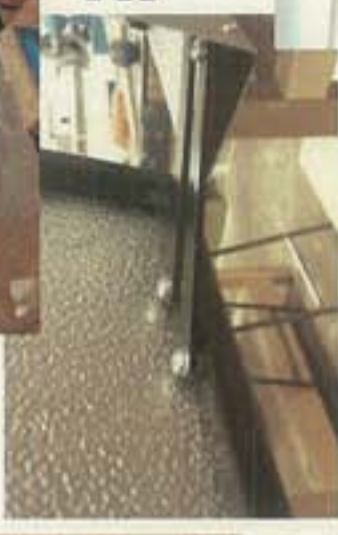
Picture of the support bars for the left hand side door.
