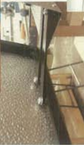
Picture of the support bars for the left hand side door.
