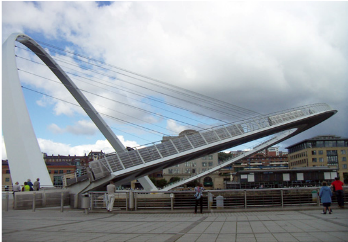
Gateshead Millennium Bridge 2002 © John Walker OCR
