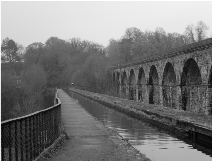
(above) The Llangollen Canal and towpath crossing the Chirk Aqueduct; the Chirk railway viaduct also runs close by
