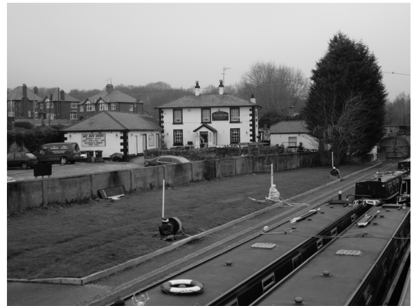
(above) A view of the Trevor Basin moorings with one of the canal-side pubs in the background – originally used by barges and quarrymen but now popular with visitors
