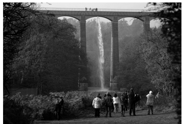
Aqueduct canal trough being emptied of water for maintenance work to take place
